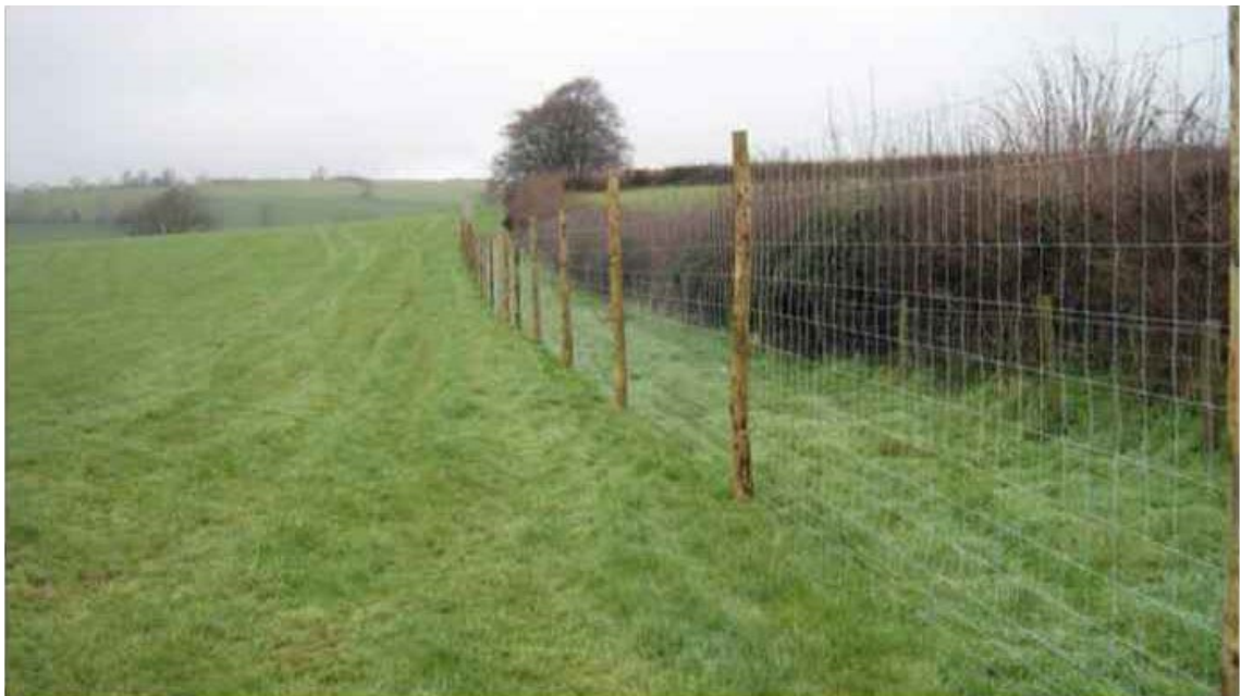
Figure 4.5: Typical Deer Fencing
